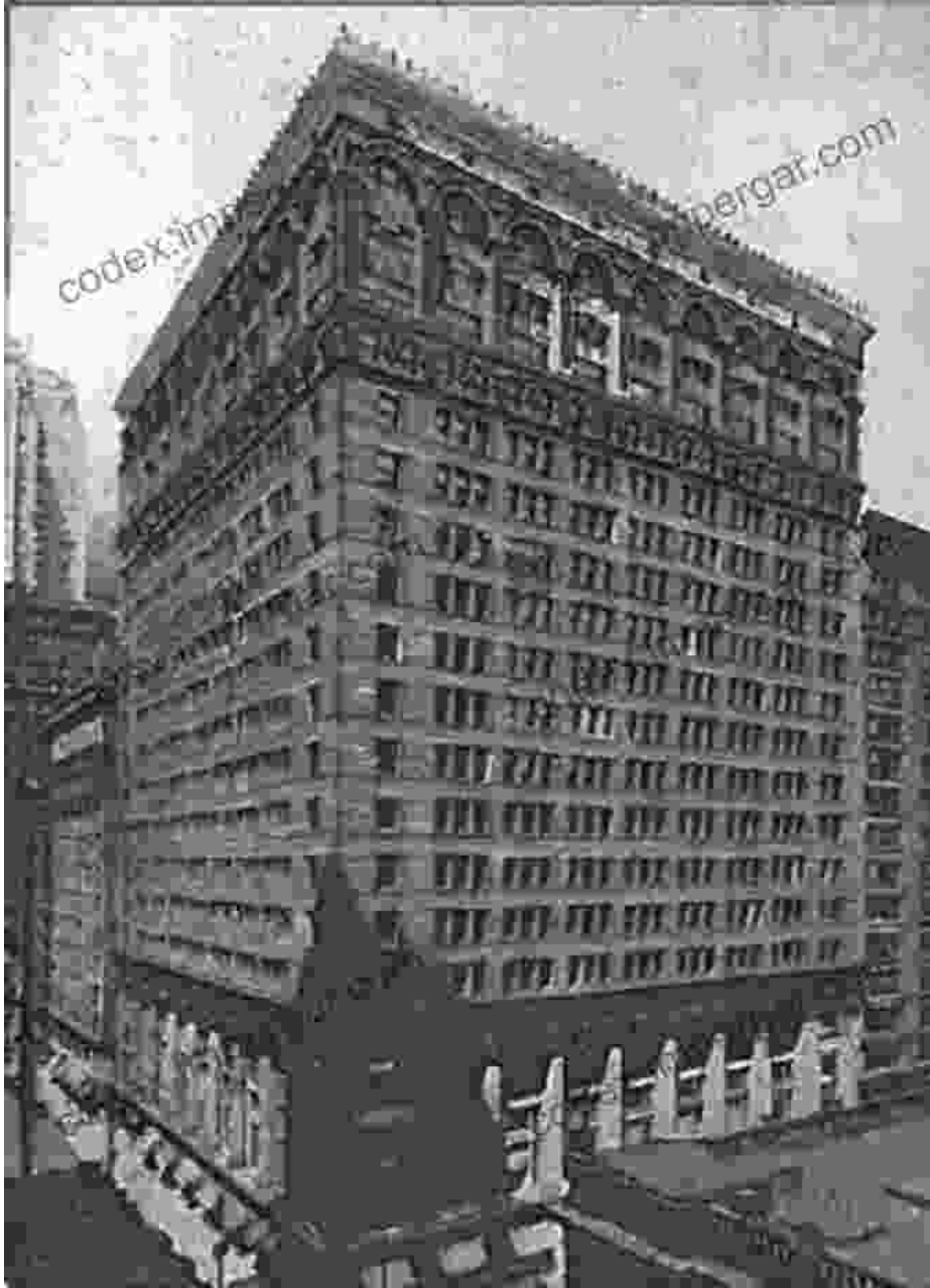
Edison Building, Rochester Downtown, circa 1930
